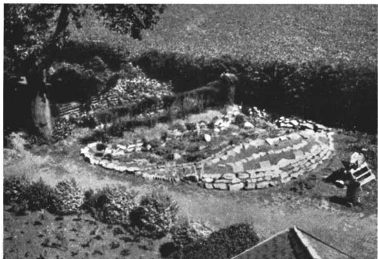
Fig. 9. —ROCK GARDEN UNDER CONSTRUCTION.
